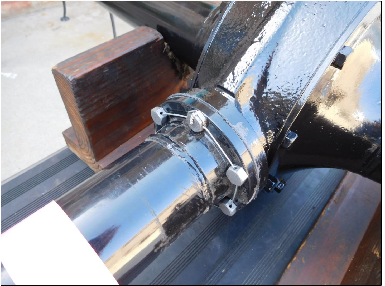
The six mounting bolts are installed and safety wired.
