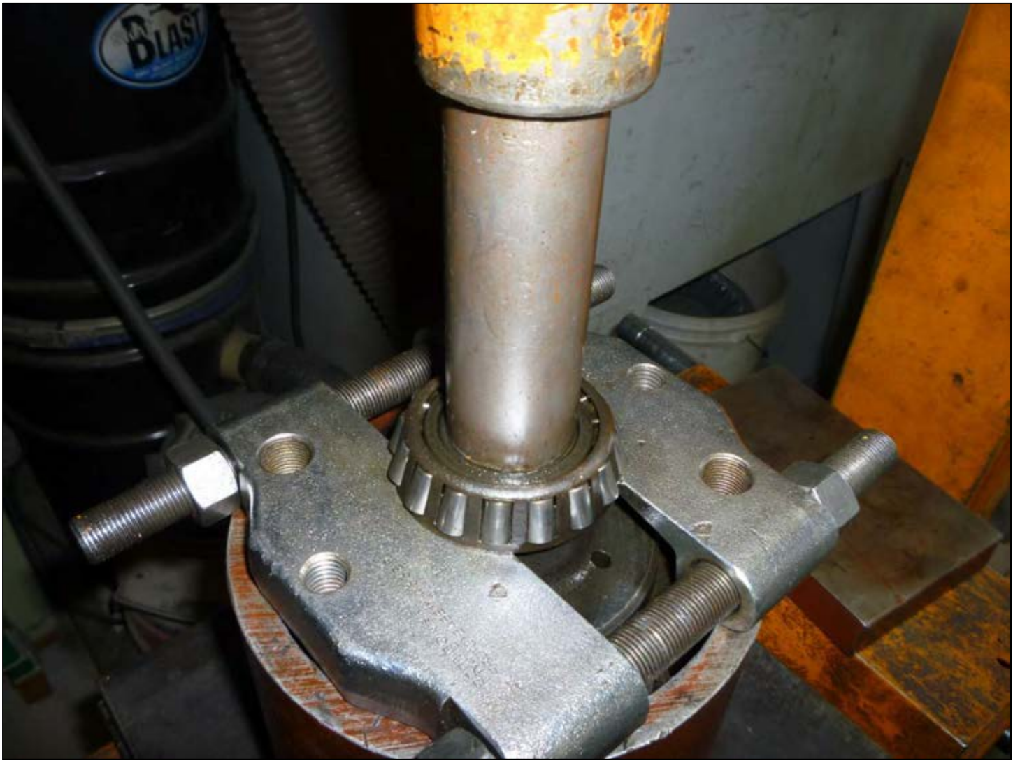
The old bearing is being pressed off the carrier half opposite the ring gear.
