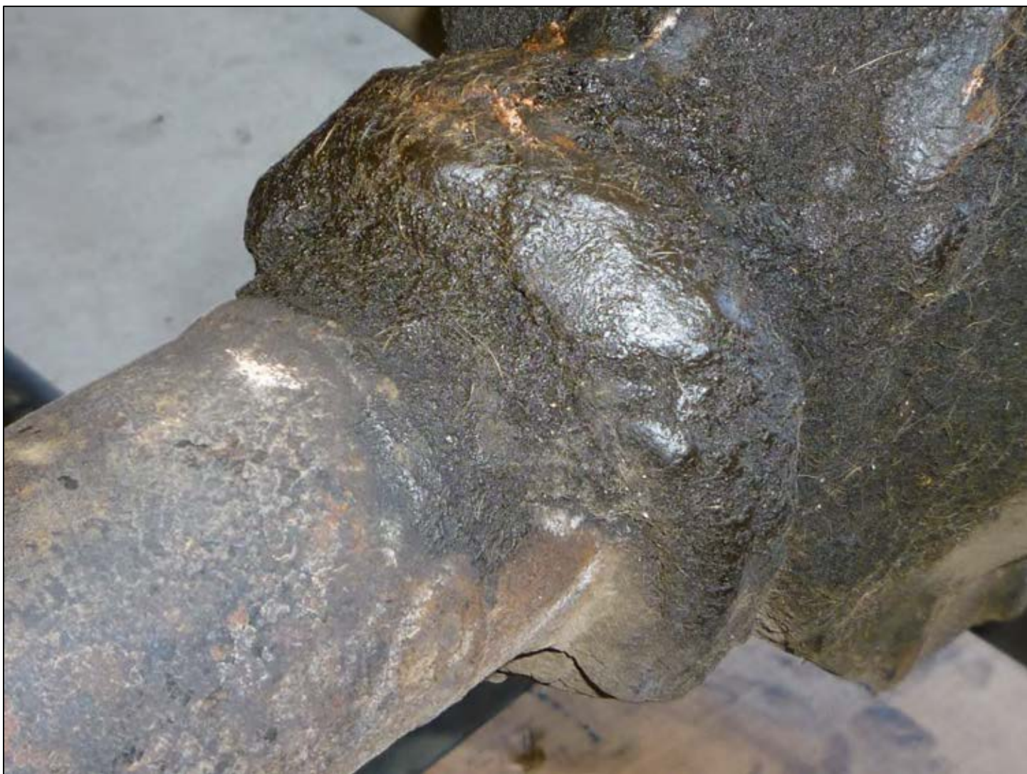
The top side of the torque tube flange is hidden in crud.
