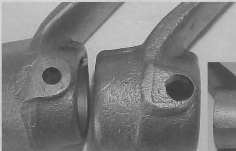
The above photo shows two A7511-B arms. The arm on the left has the original 3/16" hole. The arm on the right has been drilled out to 5/16". Note how close to the edge the new hole is.
